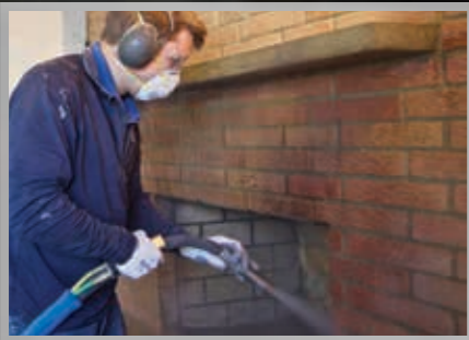
Wood and Brick Cleaning
