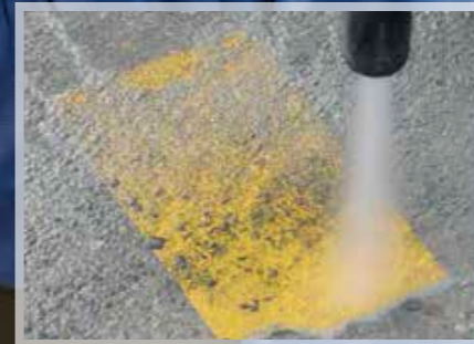
Concrete Cleaning and Surface Preparation
