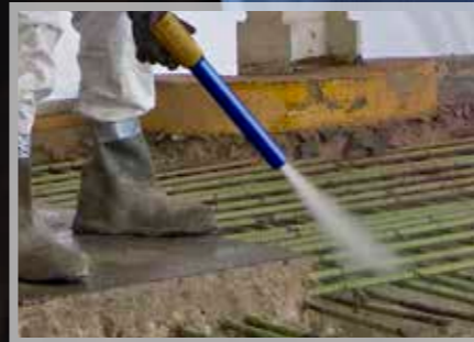
Concrete Repair and Restoration
